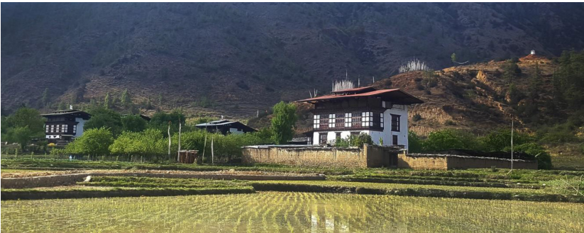
Plate 2: A traditional house in Paro, Bhutan. Note the boundary wall and also the wall of the house which is made of rammed earth. All windows are wooden and the roof which would have been of wooden shingles has been replaced by corrugated galvanized iron (CGI) sheets.
